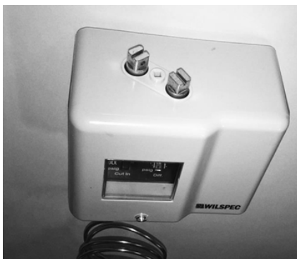
Figure 32: Adjustable Setting Screws
