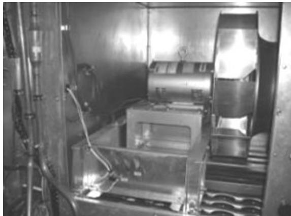
Figure 42 — 6-25 and 30 ton Supply Fan
