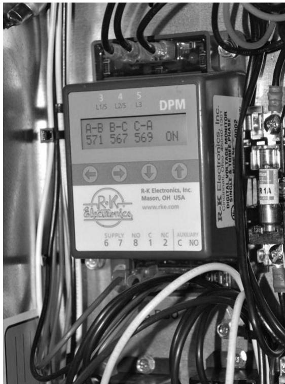
Figure 78 — Digital Phase Monitor
