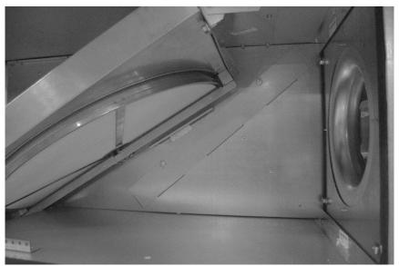
Figure 32 - H3 A or B Cabinet Outside Air Filter Access
