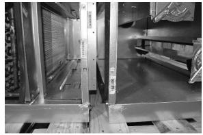
Figure 10 - Connect Sections
