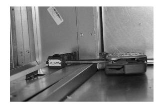
Use bar clamps or other non-destructive winching device to pull the tops of the modules together tightly.
