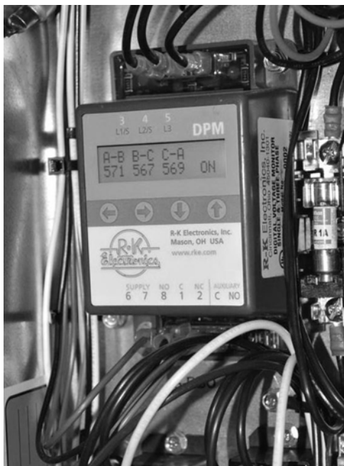
Figure 54: Digital Phase and Brownout Protection Module
