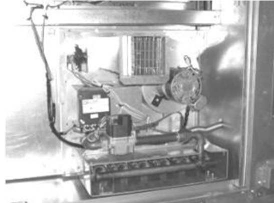
Figure 51: Gas Heat Exchanger
