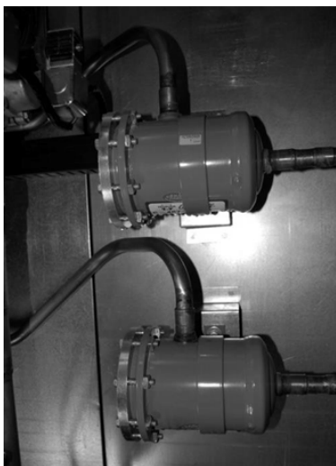
Figure 24: Replaceable Core Liquid Filters/Driers Suction Filter
