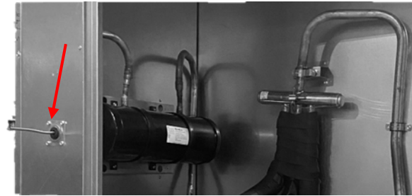
Figure 20: A2L Safety Vent Tube
