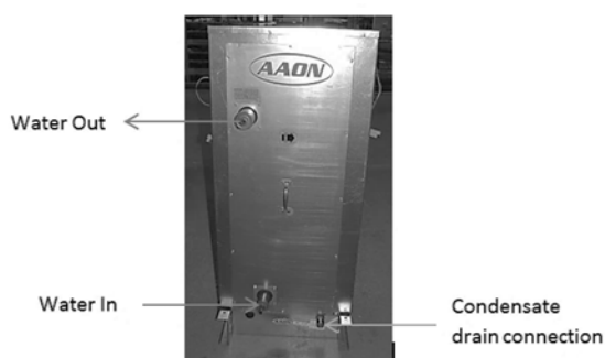
Figure 27: Chill Water Piping
