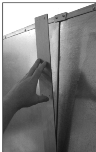
Figure 16: Strap Positioning
