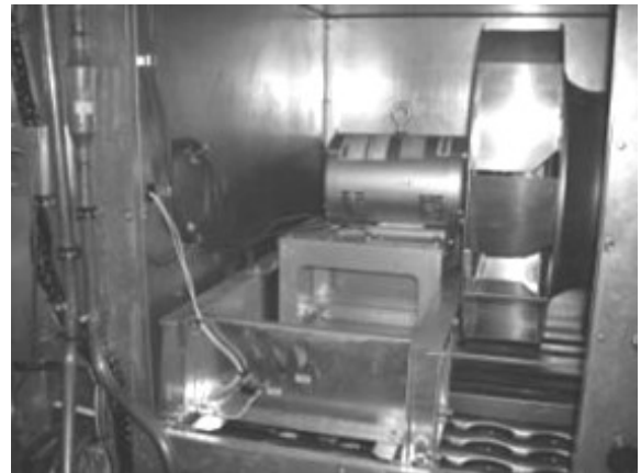
Figure 42 — 6-25 and 30 ton Supply Fan
