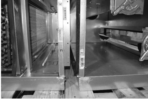
Figure 17: Connect Sections
