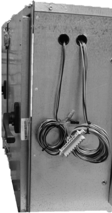
Figure 14: Low & High Voltage Quick Connect
