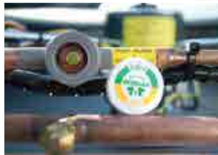
Refrigerant Circuit Sight Glass
