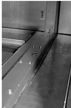
Figure 11 - Flange Overlap
