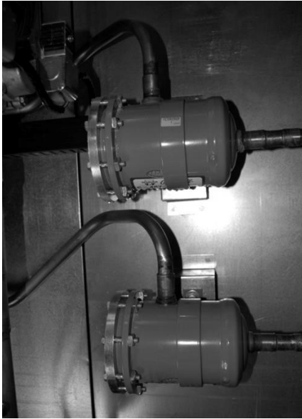
Figure 26 - Replaceable Core Liquid Filter/Driers Suction Filter
