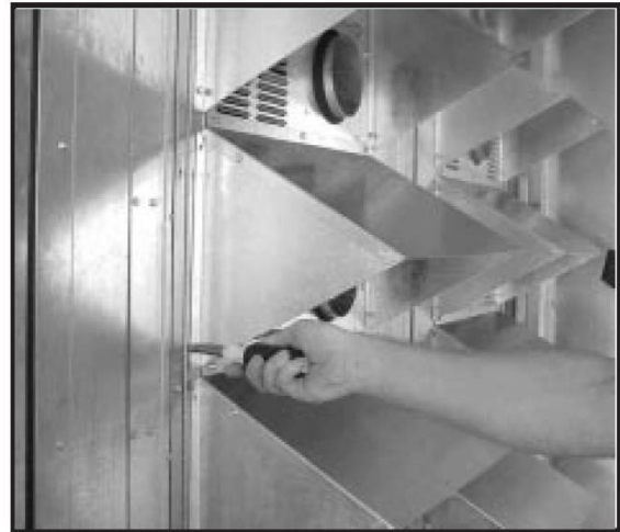
Figure 38 - Gas Heater Rain Hood Screws
