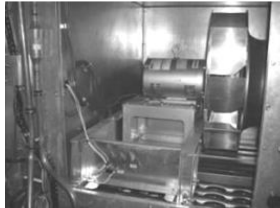
Figure 26 - 9-25 and 30 ton Supply Fan
