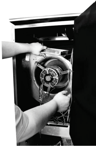
Figure 5 - Blower Assembly with Captive Panel
