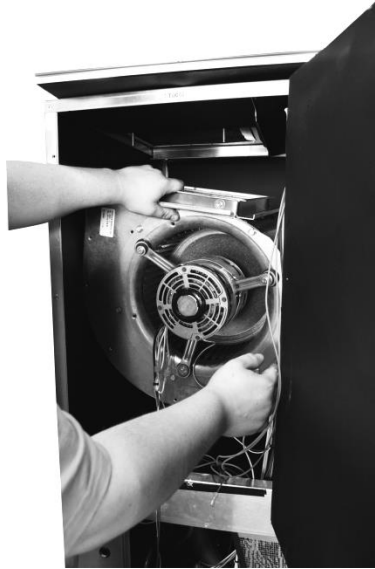
Figure 5 - Blower Assembly with Captive Panel
