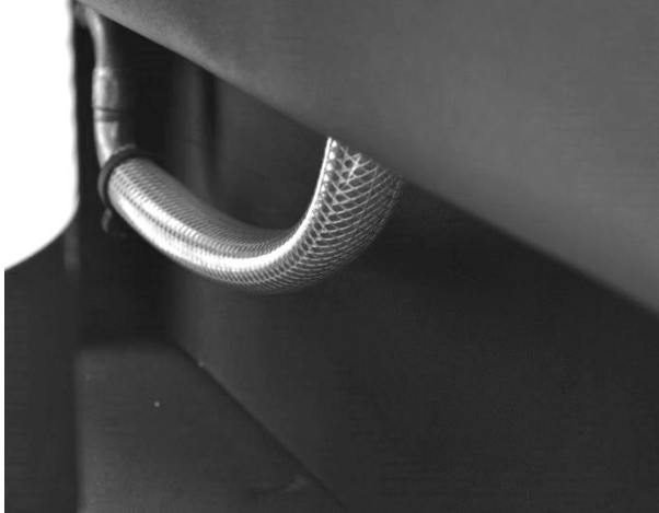
Figure 2 - Internal Condensate P-trap
