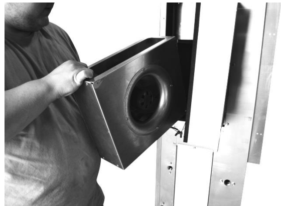
Figure 4 - Blower Assembly
