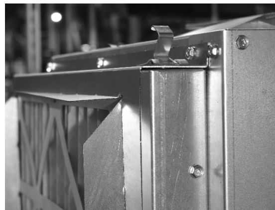
Figure 9 - Filter Rack Open with Clip
