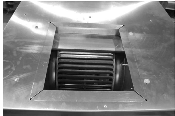
Figure 12 - Flattened Duct Flanges
