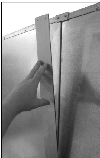
Figure 15 - Strap Positioning
