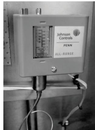
Figure 7 - Adjustable Fan Cycling Switch
