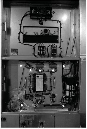
Figure 4 - Removable Internal Control Panel
