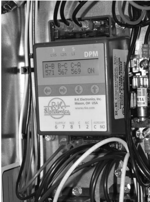
The DPM is a Digital Phase Monitor that monitors line voltages from 200VAC to 240VAC 1 $\phi$  and 200VAC to 600VAC 3 $\phi$ . The DPM is 50/60 Hz self-sensing. DPM must be wired according to unit specific wiring diagram include in the control compartment
