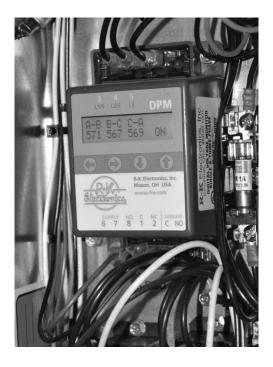
The DPM is a Digital Phase Monitor that monitors line voltages from 200VAC to 240VAC 1φ and 200VAC to 600VAC 3φ. The DPM is 50/60 Hz self-sensing. DPM must be wired according to unit specific wiring diagram include in the control compartment
