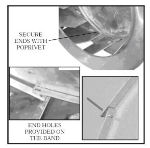
Figure 21 - Securing the Band
