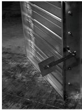
Figure 24 - Closed Back Draft Damper
