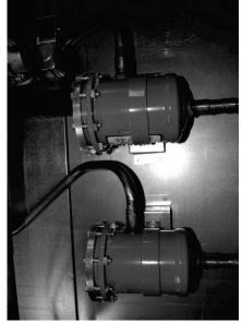
Figure 26 - Replaceable Core Liquid Filter/Driers Suction Filter
