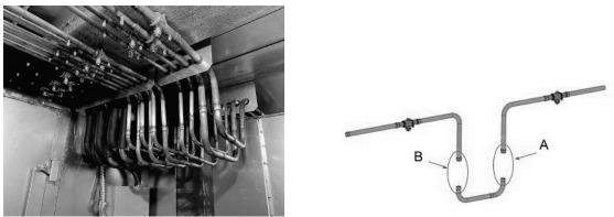
Figure 11 - Staggered assembly for refrigeration pipes
