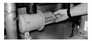
6. Replace the suction filter end plate and bolts
