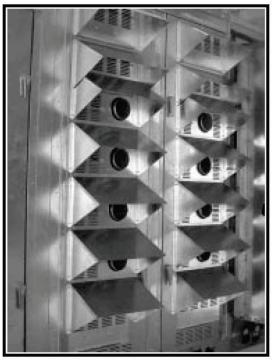
Figure 38 - Gas Heater Rain Hood
