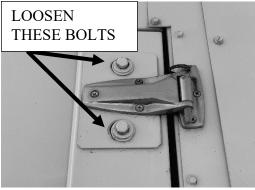
Figure 33 - Evaporative condenser access door
