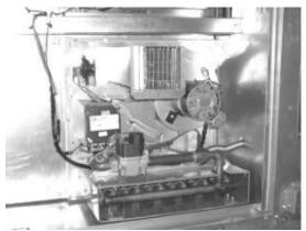
Figure 40- Gas Heat Exchanger
