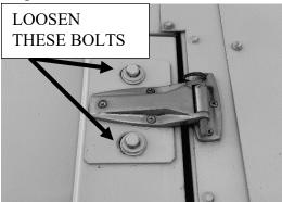
Figure 32 - Evaporative condenser access door
