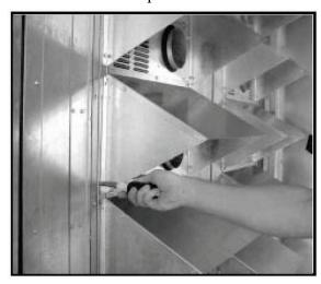
Figure 38 - Gas Heater Rain Hood Screws
