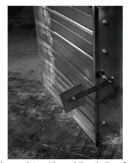
Figure 24 - Closed Back Draft Damper
