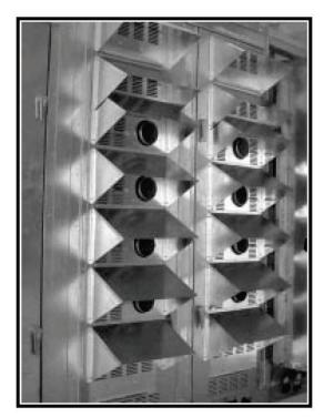
Figure 37 - Gas Heater Rain Hood
