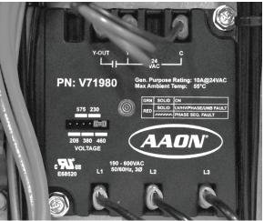
Phase and brownout module may be this type on some products (as seen in the above picture). No setup is needed with this module version, other than checking that the voltage jumper voltage matches the unit voltage
