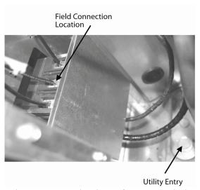
Figure 22 - Back View of Power Switch from Compressor and Control Compartment (6-50, 60, and 70 ton Units)
