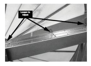
1. Loosen the three purge adjusting screws.
