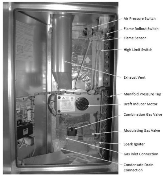
Figure 32 – Gas Heater Component Identification
