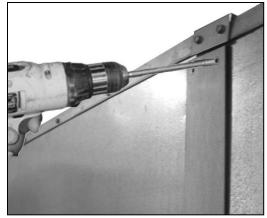
Figure 16 - Strap Installation
