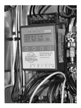
The DPM is a Digital Phase Monitor that monitors line voltages from 200VAC to 240VAC 1 $\phi$  and 200VAC to 600VAC 3 $\phi$ . The DPM is 50/60 Hz self-sensing. DPM should be wired according to unit specific wiring diagram include in the control compartment
