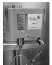
Figure 7 - Adjustable Fan Cycling Switch
