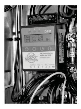
The DPM is a Digital Phase Monitor that monitors line voltages from 200VAC to 240VAC 1φ and 200VAC to 600VAC 3φ. The DPM is 50/60 Hz self-sensing. DPM shall be wired according to unit specific wiring diagram included in the control compartment
