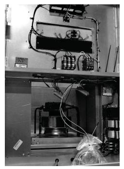
Figure 5 - Supply Fan Access after removing control panel
