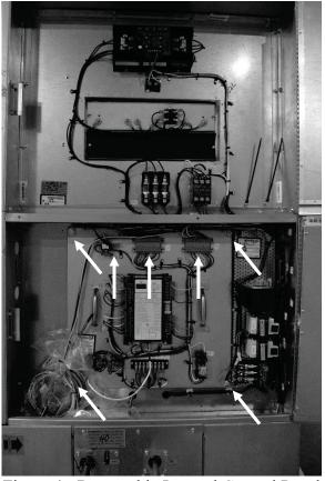
Figure 4 - Removable Internal Control Panel
