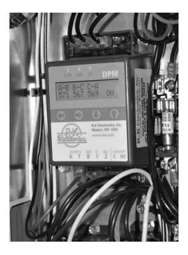
The DPM is a Digital Phase Monitor that monitors line voltages from 200VAC to 240VAC 1φ and 200VAC to 600VAC 3φ. The DPM is 50/60 Hz self-sensing. DPM should be wired according to unit specific wiring diagram include in the control compartment
