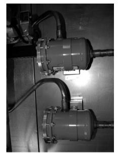
Figure 26 - Replaceable Core Liquid Filter/Driers Suction Filter
