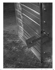
Figure 24 - Closed Back Draft Damper
