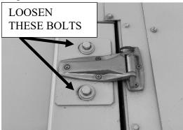
Figure 32 - Evaporative condenser access door
