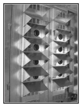
Figure 37 - Gas Heater Rain Hood
