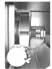
Figure 26 - 2-6 ton Supply Fan
