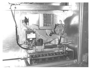
Figure 37 - Gas Heat Exchanger
