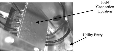
Figure 19 - Back View of Power Switch from Control Compartment
