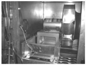
Figure 38 - 11-25 and 30 ton Supply Fan
