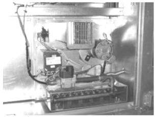
Figure 23 - Gas Heat Exchanger
