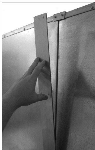
Figure 15 - Strap Positioning
