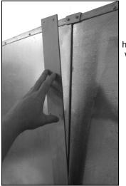
Put straps in position, hold in place and attach with self-tapping sheet metal screws.
