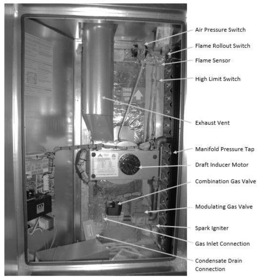
Figure 32 – Gas Heater Component Identification
