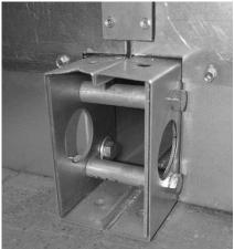
Figure 10 - Bolted Base Rail
