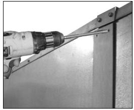
Figure 16 - Strap Installation
