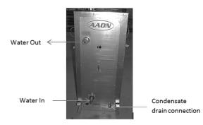
Figure 25 - Chill Water Piping
