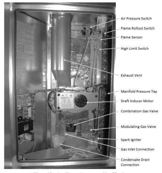
Figure 32 – Gas Heater Component Identification
