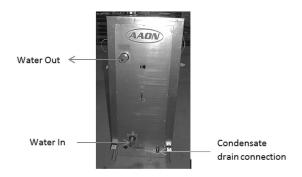
Figure 25 - Chill Water Piping
