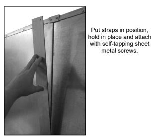
Figure 15 - Strap Positioning
