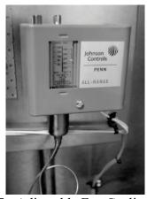
Figure 7 - Adjustable Fan Cycling Switch
