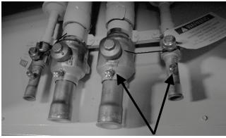
Figure 5 - CU evacuation connections
