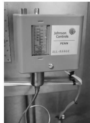
Figure 8: Adjustable Fan Cycling Switch
