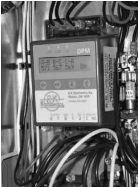
The DPM is a Digital Phase Monitor that monitors line voltages from 200VAC to 240VAC 1 $\phi$  and 200VAC to 600VAC 3 $\phi$ . The DPM is 50/60 Hz self-sensing. DPM should be wired according to unit specific
