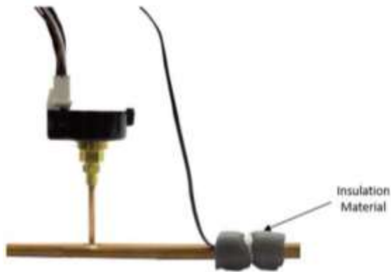
Figure 17 - Insulation secured to the thermistor
