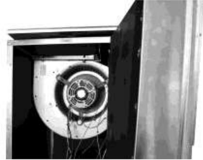
4) Grip the blower assembly with both hands and pull it about  $\frac{1}{2}$ " or until it clears the captive panel at the assembly.
