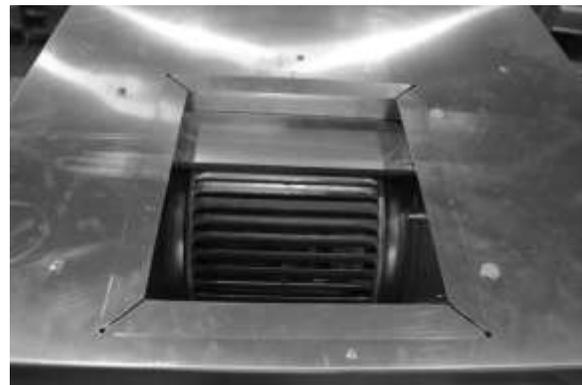
Figure 10 - Flattened Duct Flanges
