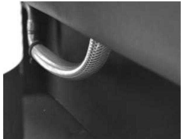
Figure 2 - Internal P-trap
