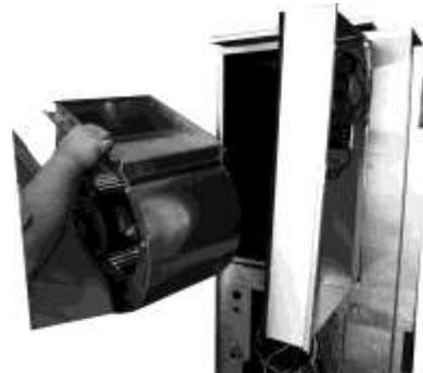
Figure 6 - Blower Assembly, Shown Pulled Away From Blower Panel
