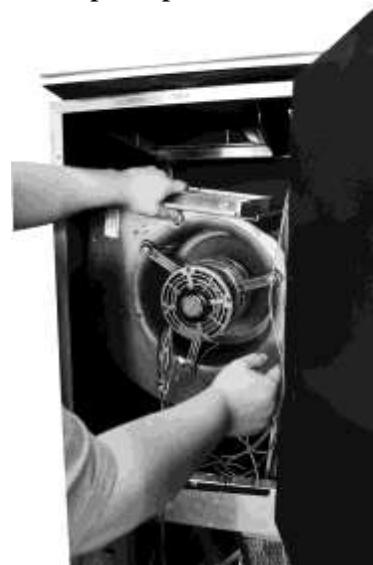
Figure 5 - Blower Assembly with Captive Panel
